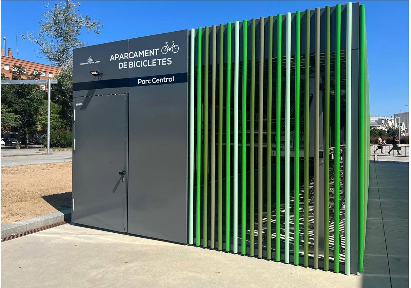
In Girona's Parc Central, next to the high-speed train station, the bus station and close to the Renfe train station, a parking area with a capacity for 70 bicycles has been installed. It is made of a metal structure based on coloured laminated profiles and is designed to be flexible so that it can be expanded or reduced, or moved to another location if required in the future..
