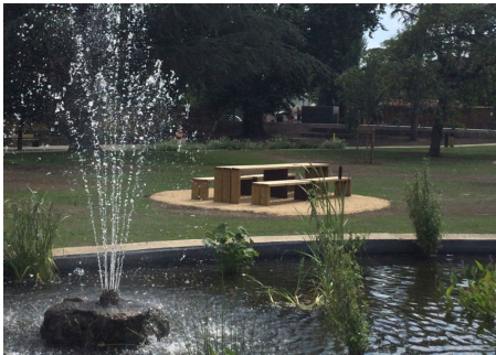
Installation of Gavarres benches, tables and bins, ideal for rural environments thanks to the use of wood and Corten steel.
