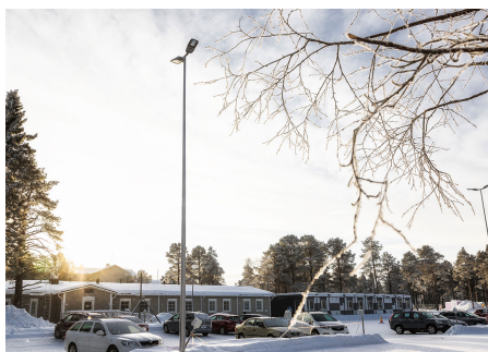
Milan luminaires and floodlights for the renovation of the lighting system using energy-efficient LED technology in the new educational centre in Inari.
