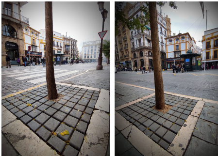
Ecological grate made of recycled plastic for Seville's trees.
